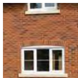
Flat gauged arch - segmental
