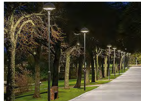
Fig. 29: Pedestrian column lighting
