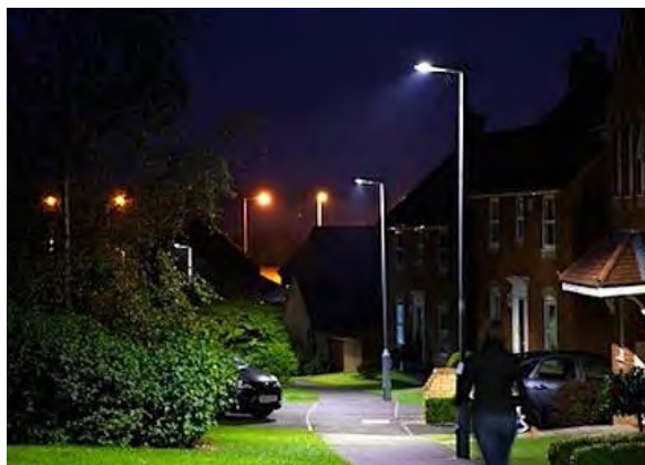
Fig. 28: Street column lighting
