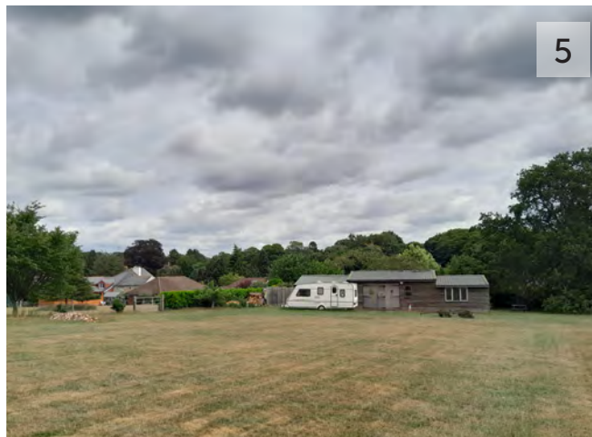
Photograph of storage shed located on eastern boundary of Site - to be demolished
