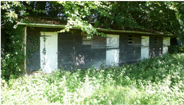
Photo 15: view showing the timber stable block building in the north-western corner of the site.
